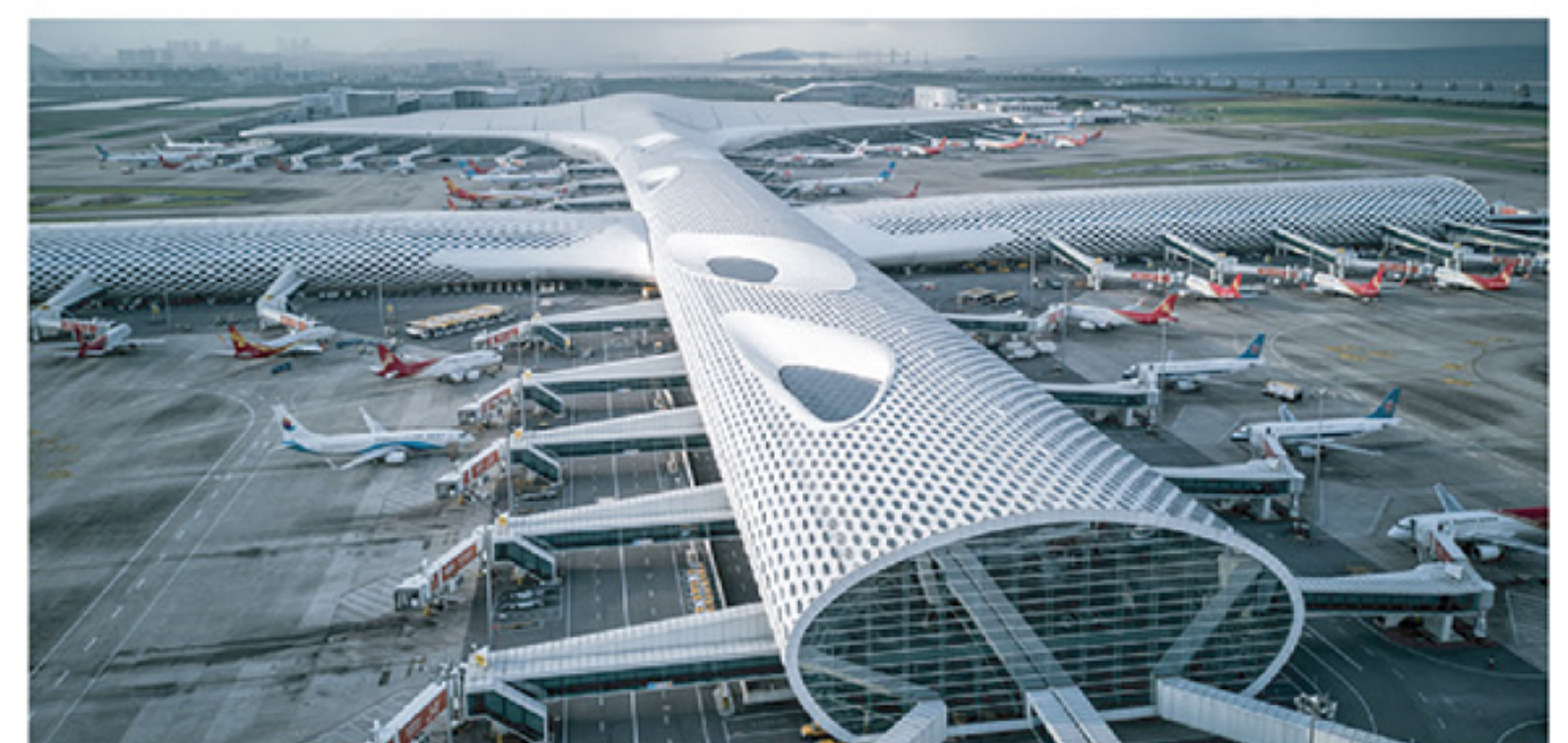
Shenzhen Bao'an International Airport Satellite Hall
